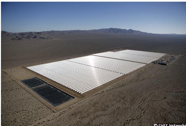
Figure 6. Nevada Solar One, parabolic mirror array, which truncates ephemeral drainages, including a large wash visible at nearest corner of array. Note that surface features and vegetation were eradicated within the array's footprint
